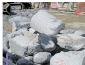
Pieces of rock extracted with the bored pile.
