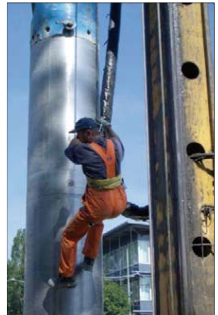
The use of a rubber loader as a "working platform" and safety harness are examples of inadequate means of access
