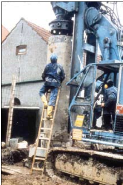
Screwing and fastening the column casing to the driver using a ladder
